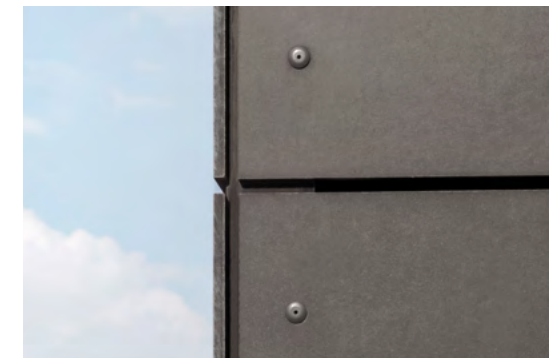
Visible mounting of the fiber cement panels with colored rivets
