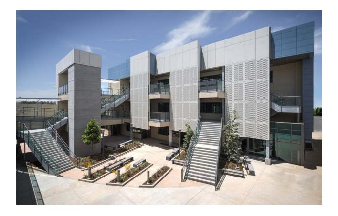
An integral part of a comprehensive sustainability strategy aimed at LEED Gold certification, the architects devised a rain screen facade clad in Swisspearl panels, which will boost the building's energy performance and help keep long-term maintenance costs to a minimum.
