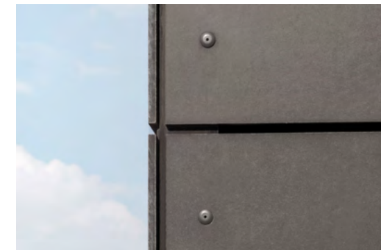
Visible mounting of the fiber cement panels with colored rivets
