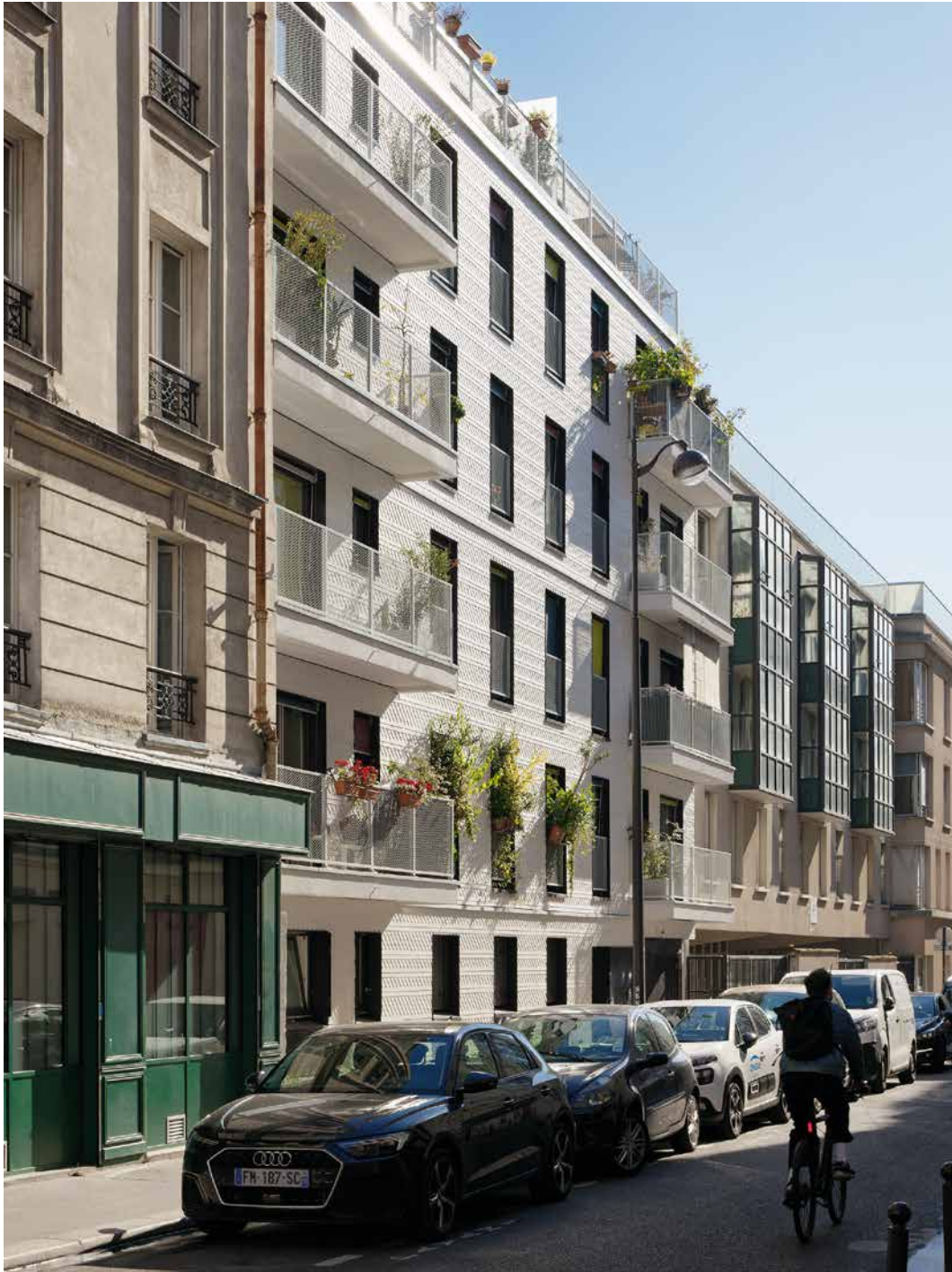
The social housing project from the 1980s was renovated and refurbished for energy efficiency. The new exterior thermal insulation is clad in small, white fiber cement shingles. Brightly colored sun blinds set bold, cheerful accents.
