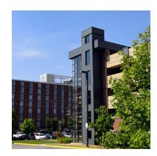
Ceramic5 porcelain panels with a concealed F1.40 fastening system were selected as the featured cladding on this addition to an existing parking garage at Purdue University.
