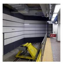
Cooper Carry of NYC designed the first new subway in NYC, with a Ceramic5 engineered porcelain stone cladding solution provided by Cladding Corp. Ceramic rainscreen systems are becoming more and more popular in the architectural design community. System Type: F1.40 Panel Type: Ceramic5 Architect: Cooper Carry - NYC Installer: Judlau Contracting Completed: 2009
