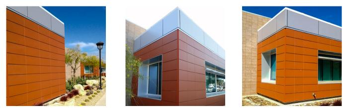
Terra5 was a natural choice for GKK Works of San Diego for the new Miramar College Service Center. The terracotta rainscreen added warmth and was the featured architectural facade material. Various features were added to create this energy-efficient building – including the use of green sunscreens. System Type: F2.22 Panel Type: Terra5 Architect: GKK Works Installer: Sun Pacific Glazing Completed: 2011
