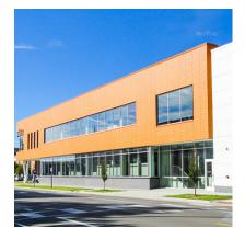
Intermec Offices of Cedar Rapids used the Terra5 TC18 terracotta panels and the complementary sunscreen baguettes on their new facade designed by OPN Architects. The simple clean lines with beautiful terracotta makes heads turn to see this new facade. System Type: F2.22 Panel Type: Terra5 Architect: OPN Architects Installer: Midwest Glazing Completed: 2011
