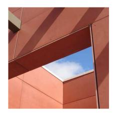
A high-performance, state-of-the-art, green fieldhouse facility in San Diego, complete with a drained and back ventilated System5 rainscreen by Cladding Corp. The higher education building was designed by Carrier Johnson of San Diego and incorporated Concrete5.
