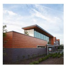
RDG Planning and Design of Omaha designed a HPL rainscreen wall featuring Plus5 substructure. An exposed fixing system was used and the depth accommodated fiber insulation. System Type: F1.10 Panel Type: HPL
