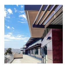
Baker Nowicki Design Studio designed the new Technology Magnet School in Escondido, CA called Del Lago Academy. Ceramic5 in two colors were used incorporating a visible clip attachment system. The 19,000 square feet of ceramic tiles were in 2 foot by 4 foot sizes.
