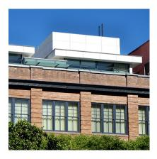
FME Architecture and Design designed a stunning roof top private club in San Francisco called The Battery. White fiber concrete panels were installed with Plus5 sub-structure. The adjustable and concealed anchor system created for a beautiful facade.
