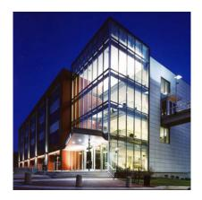
Towson University's 7800 York Road – Technology Building integrates terracotta and ceramic rainscreen. The Ceramic5 used an elegant, crisp white panel in a stacked bond pattern. The F1.40 system is a concealed attachment sub-structure.
