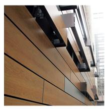
FXFowle Architects of New York City designed the Hudson Hill Condominiums at 462 West 58th Street using a Plus5 attachment system for HPL panels. The Plus5 sub-structure was selected to allow for an interesting design – the walls move in and out to create a stunning facade.
