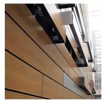
Group Goetz Architects had the responsibility to upgrade and reclad the entrance of 2131 K Street in Washington, DC's "Golden Triangle" area. Dark-grey fiber concrete panels were installed with Plus5 substructure. The adjustable system allowed the architect to install the panels with minimal cavity depth.
