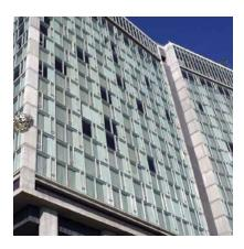
Straddling the High Line, NYC's newest iconic landmark, The Standard Hotel, is now complete with a Concrete5 engineered rainscreen system from Cladding Corp. Ennead Architects were the designers.
