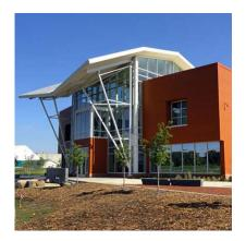
LHB of Minneapolis designed the new Cascade Meadow Wetlands Center which requires 55% less energy than code. Cem5 and System5 were used to contribute towards the buildings energy efficiency. The Hci.10 substructure was installed on an ICF wall.
