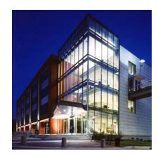
Towson University's 7800 York Road – Technology Building integrates terracotta and ceramic rainscreen. The Ceramic5 used an elegant, crisp white panel in a stacked bond pattern. The Vci.40 system is a concealed attachment sub-structure.
